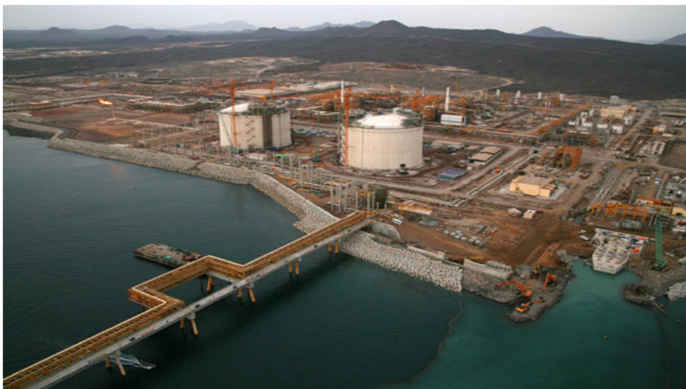
Photo of the project of liquid natural gas, Balhaf, the coast of Shabwah, Eastern Yemen. 5
